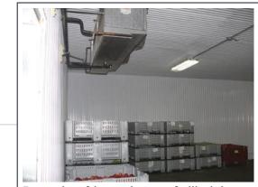
Ensure the refrigerated storage facility is insulated and sealed to prevent the entry or escape of air and provide good air distribution within the storage.
