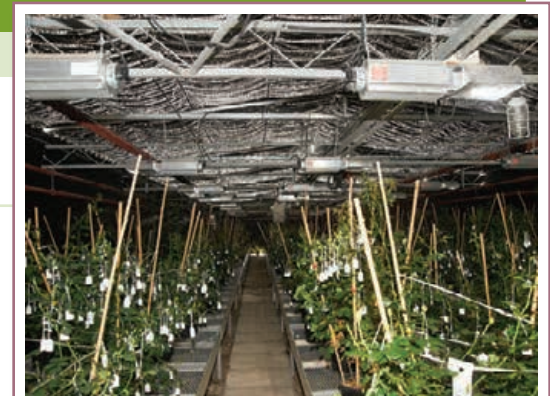
Black-out screening will reduce the offsite impact of night-time lighting.
