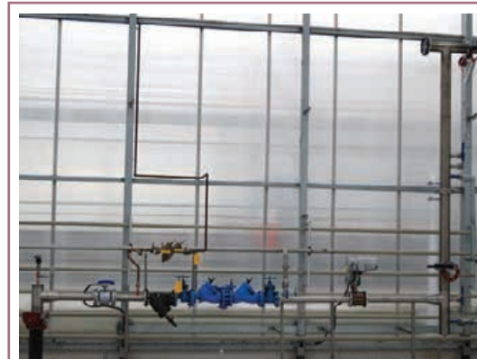
Whenever fertigation equipment is used, always check that anti-backflow devices are installed and operating properly to prevent any backflow contamination of the water system.
