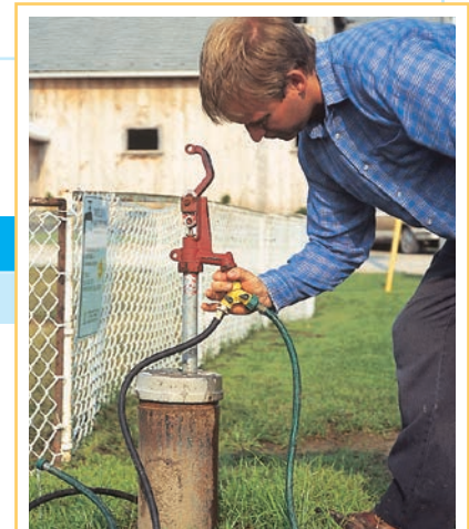
This drilled well metal casing has a frost-free hydrant faucet with an anti-backflow device.
