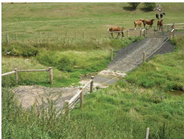
A fenced, bed-level crossing will manage livestock impact on the watercourse while providing access to pastures.
