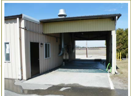
A dedicated mixing/loading area will reduce the risk of surface or ground water contamination.
