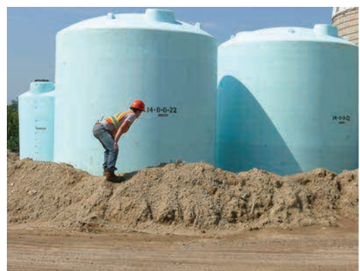
Scheduled monitoring of both the storage and the containment area reduces the risk of loss of material.
