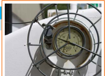
A vacuum reading indicates that both walls of a double-walled tank are sealed.
