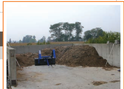
If the compost pile will be mixed and emptied with a loader, a concrete floor is preferred for ease of use, cleanliness and runoff management.
