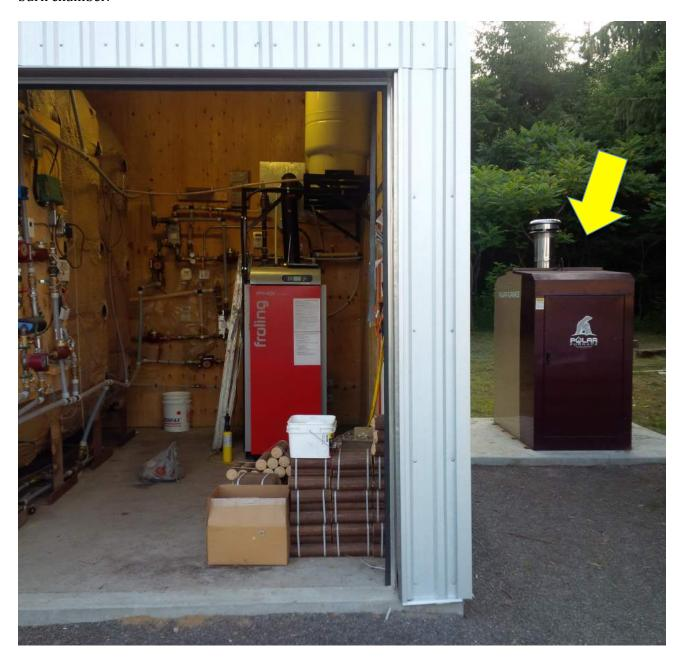
Based on the manufacturer's calculation examples, the firebox allows the operator to load wood twice a day to sufficiently heat a normal size house and provide some domestic hot water. The secondary burn chamber allows the reintroduction of secondary combustion air to combust unburnt wood gases or smoke before it exits the heating appliance. A large bright yellow flame is
